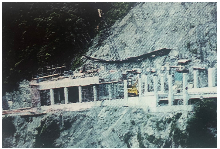
Construction of a rock fall protection structure
