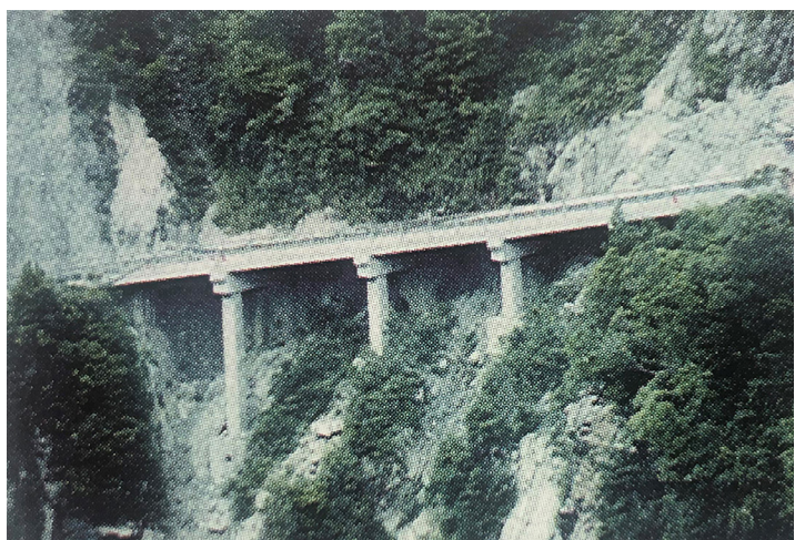
Cantilevered section of roadway approaching the viaduct
